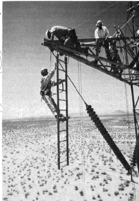
Figure 9.20. Installing vee arrangement of suspension insulator strings carrying four bundled conductors per phase at 300 kV. (Courtesy of Ohio Brass Company.)
