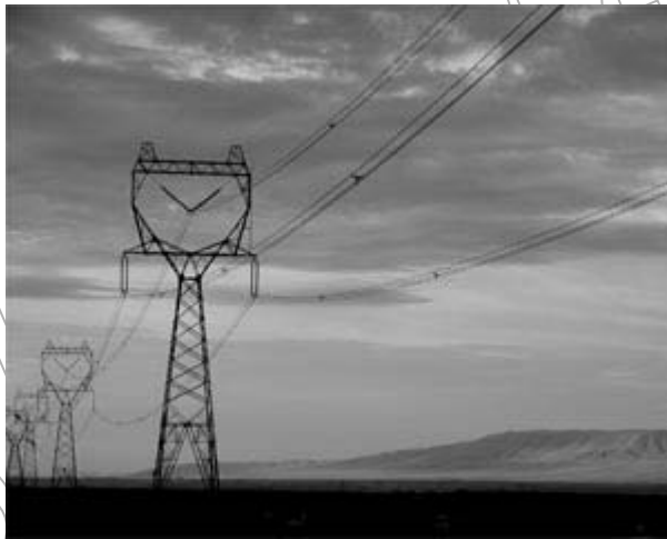
Torre Semiflexible de Acero, 500 kV. Arkansas Power and Light Company
